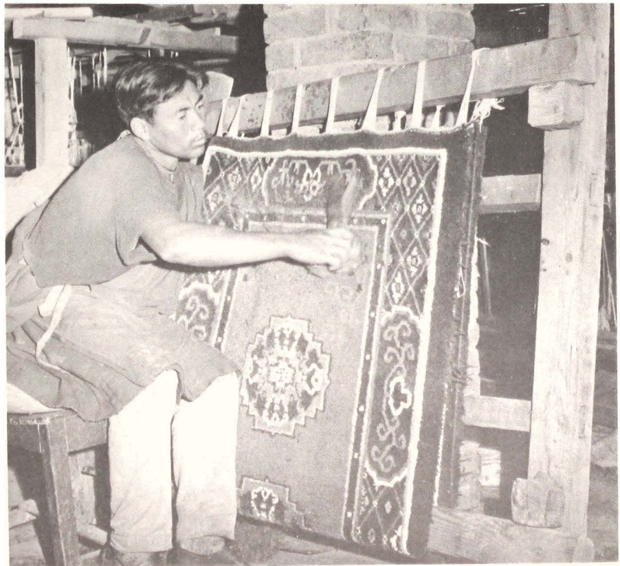
fig. 56. Shearing a carpet on the loom.
